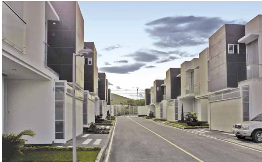
X-Caret Constructor: Odicco Cúcuta
